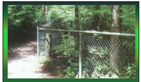
Fencing Separates an RMA from a Heavily Used Trail
