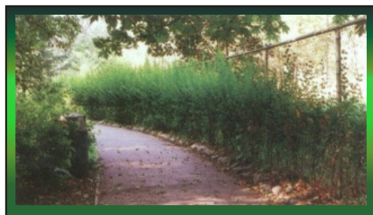
Combination Fence with Vegetative Barrier
